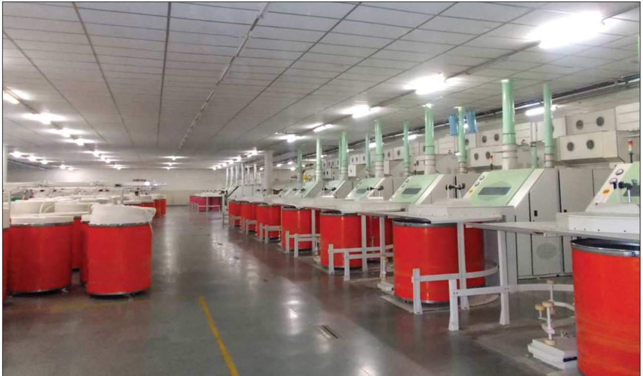
View of Spinning Plant, VPL Nalagarh
